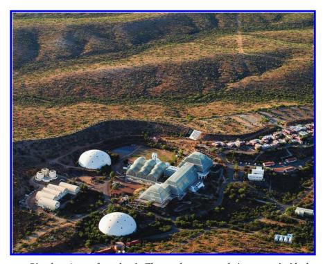
Biosphere 2, seen from the air. The two domes control air pressure inside the main structure, a collection of connected buildings that contains a large soil experiment, a rainforest, and a scale-model ocean. Photograph: Fred Powledge (with thanks to pilot Sandra Lanham, Environmental Flying Services).
